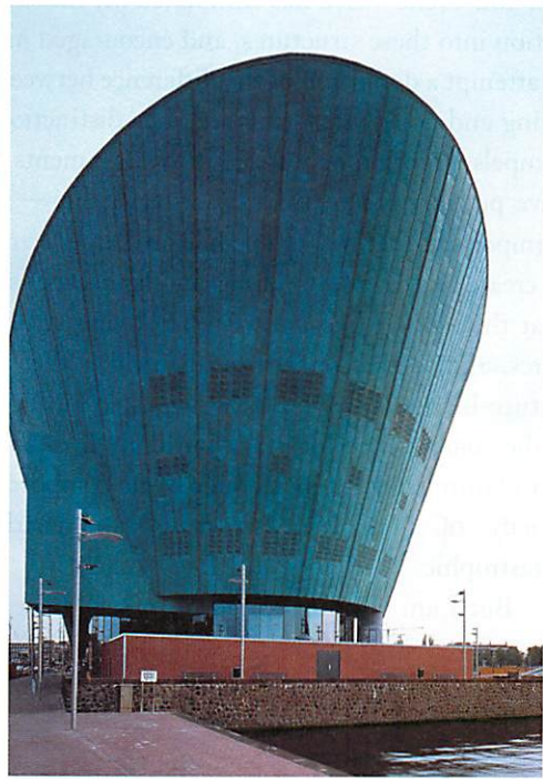
Non-living structure: Technology center, Amsterdam
